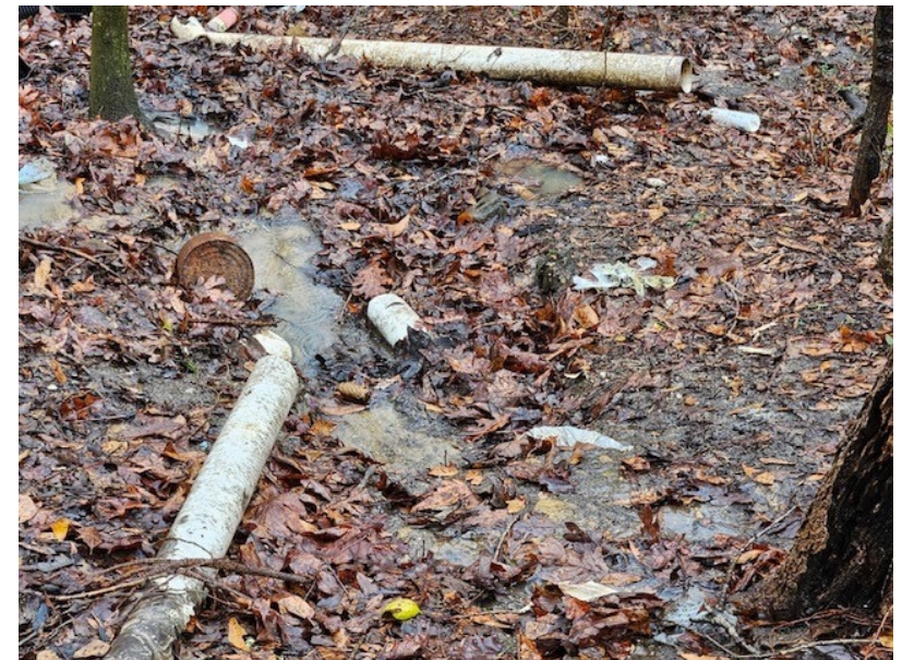
Straight Pipes and Raw Sewage Discharge
